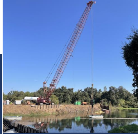
Stockton East Water District Bellota Weir Mods
