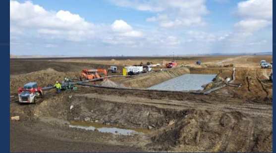
Rapid Disaster Infrastructure Repair Rockport, Missouri
