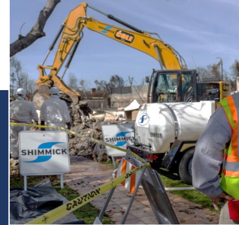
Palisades Fire Cleanup
