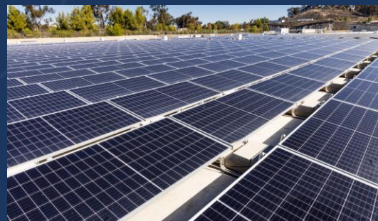
Miramar Reservoir Pump Station Improvement Project San Diego, California
