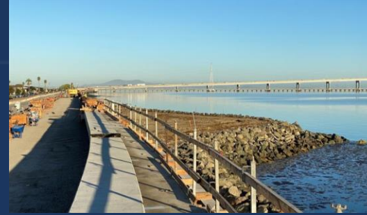
Foster City Levee Improvement Foster City, California
