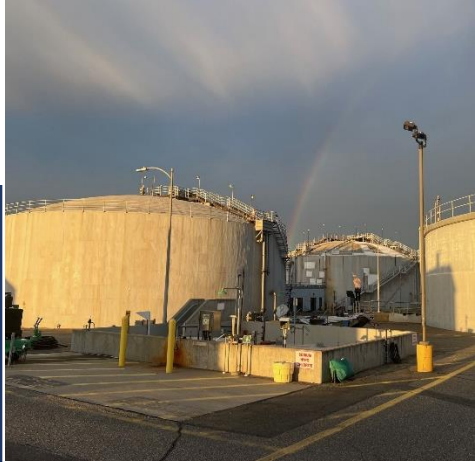
City of Modesto River Trunk Pump Station Project
